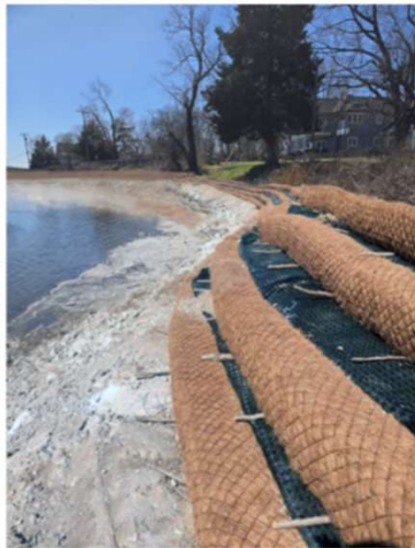
← Extending shoreline Gentler topography Hay or other locally-sourced material as anchor
