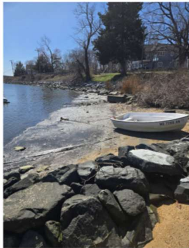
Existing conditions 1:2 slope at edge
